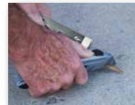
5. Gun Slab into the crack. For wider cracks (1" wide or more), apply 3 beads: 1 on each side of the crack, and another down the middle. This ensures enough product is in the joint, and makes tooling easier.
