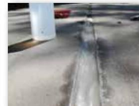
Slightly recessed Slab bead after cure
